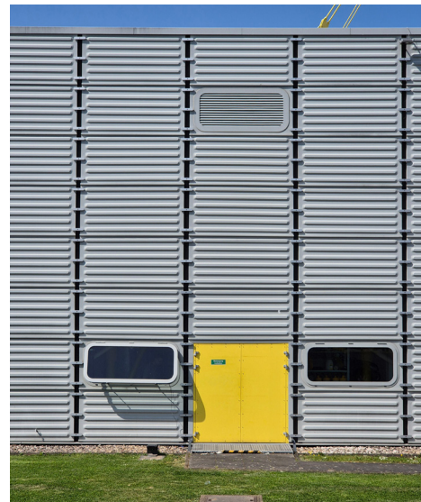
The Igus Factory by Grimshaw, in Cologne, Germany (2000) exemplifies adaptable building skins through a system of interchangeable panels - closed, louvered, glazed, and service ready - that allows quick modifications and expansions. For this study, it serves as a key precedent in adaptable envelope design, with attention to how similar strategies might be realized using localized and low-emission materials.
