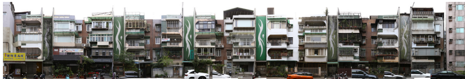
Figure: The southside of Alley 6, Lane 137, Sec. 5 Minsheng East Road (民生棟樓五段6巷137弄) in the Songshan district of Taipei, Taiwan. A standardized concrete building, with six stairwells, each with three units on either side (not counting the ground floor) which are mirrored identical, totalling 36 identical units. After the user's interventions, not two units are any longer the same. © Digital photo collage by author, 2025.
