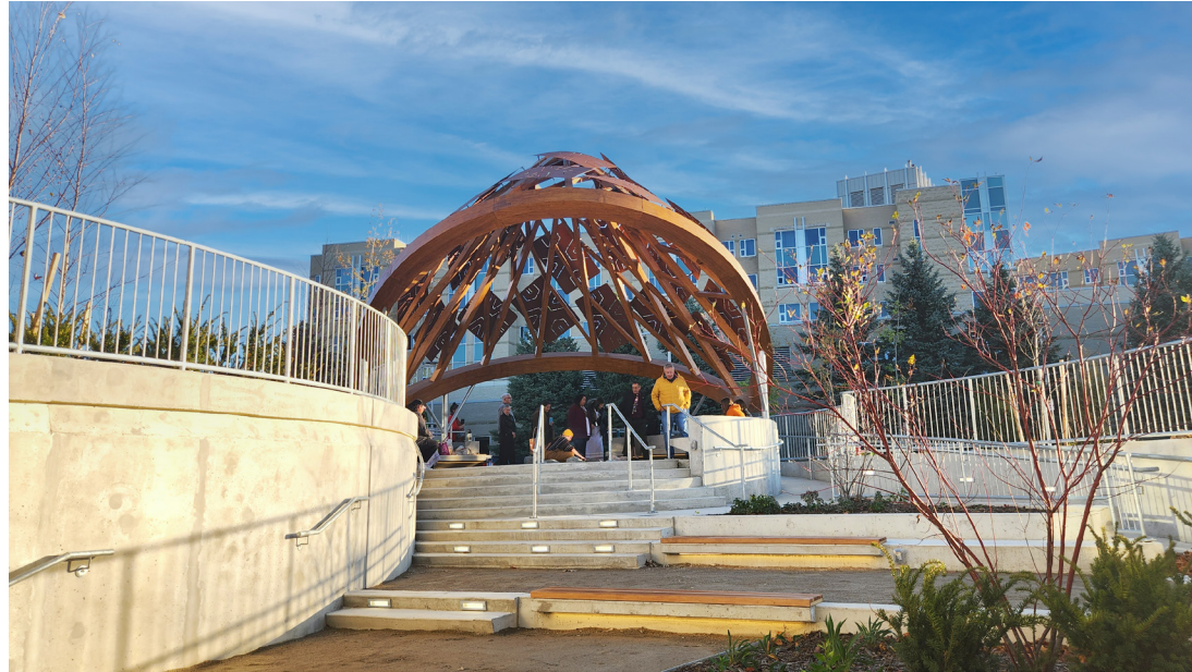
The Wampum Learning Lodge (completed in 2022), Western University, London, ON, Canada. Project by Tillmann Ruth, Robinson Architects. Design Team: Wanda Dalla Costa, Dolores Tierra Miller and Rocky Hanish Cremonini. Image courtesy of the design team.
