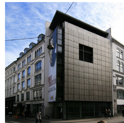
B.T. House, 8 Kristen Bernikows Street, Grønnegade, Copenhagen by Henning Larsen (1994). © Photo by Robert Lemon.
