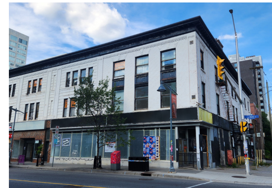
227 Bank Street, Ottawa, Ontario, Canada, built in 1888. Tenants were fully evicted in 2025 in preparation for redevelopment. Image by author.
